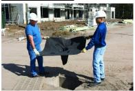
The Ultra-Drain Guard is made from a polypropylene geotextile and keeps sediment, hydrocarbons and other pollutants out of the Stormwater system. The large sediment accumulation pocket holds up to 18kg of silt, sediment and rubbish as well as 3,5 litres of oil and grease. The built-in overflow ports avoid flooding in heavy rain events.
