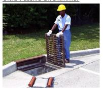
The Ultra-Passive Oil Skimmer is made of unique polymer absorbent and bonds oil to the polymer matrix to prevent leaching. It will not create ponding or clog due to sediment. Each unit hold up to 8 litres of oil and the ties allow the unites to be connected to each other or to grates to stop them disappearing down the drain.
