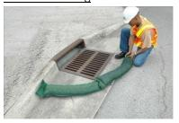
The Ultra-Gravel bag is made from tough UV resistant polymer material so it lasts and can even be driven over. It can be used for erosion control, basic Stormwater protection and more. It simply closes by using cable ties and it can be filled with gravel or other aggregate.
