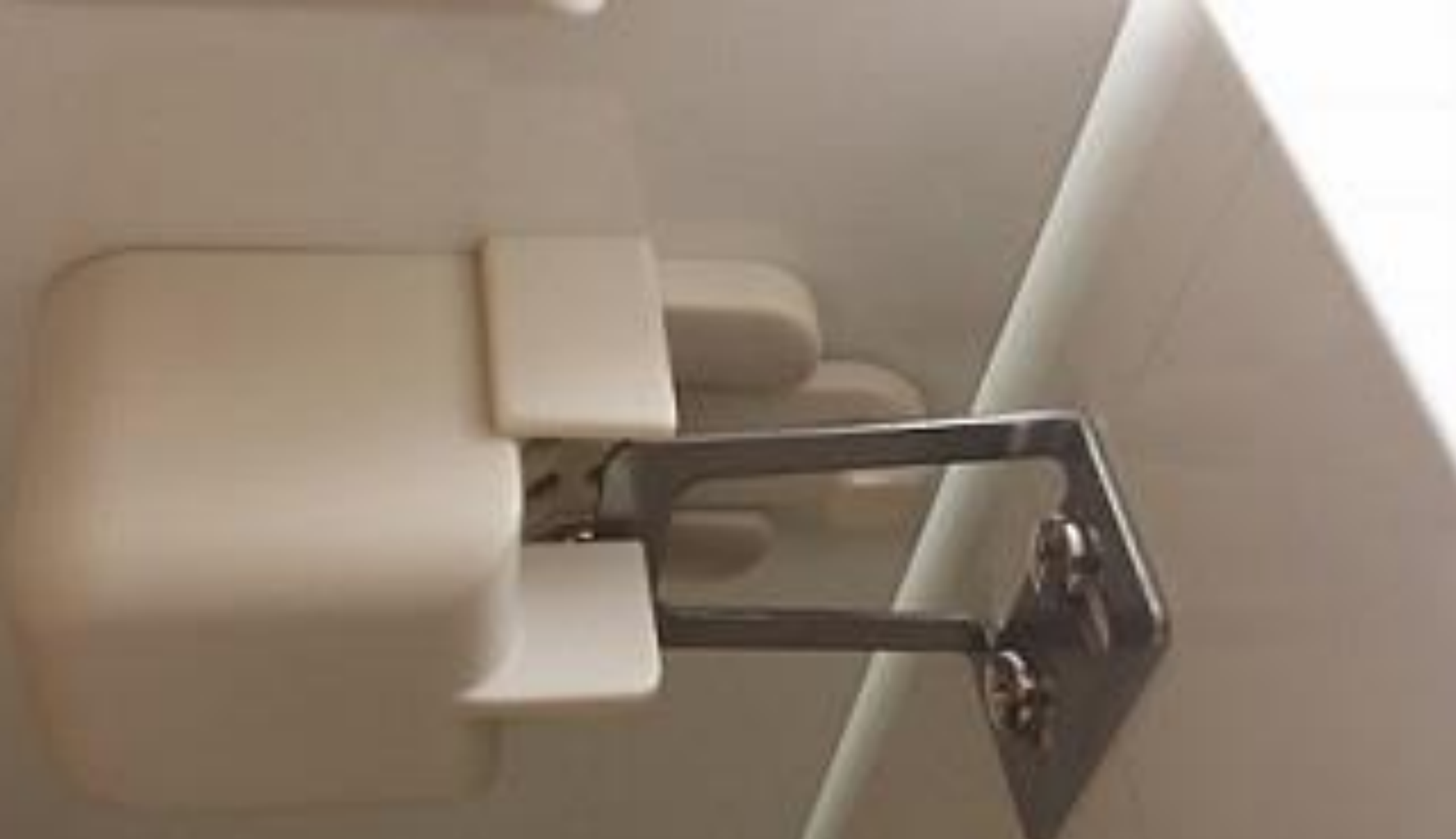
Earthquake Sensing cupboard latches
